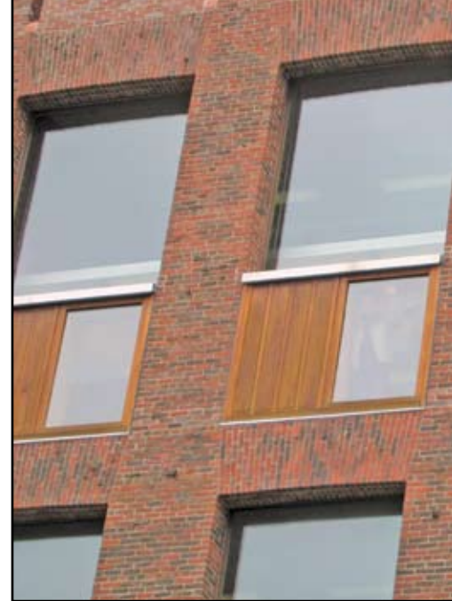
Tapered ends of the brickwork at the column and spandrel intersection. Courtesy of Steven Szycher.
