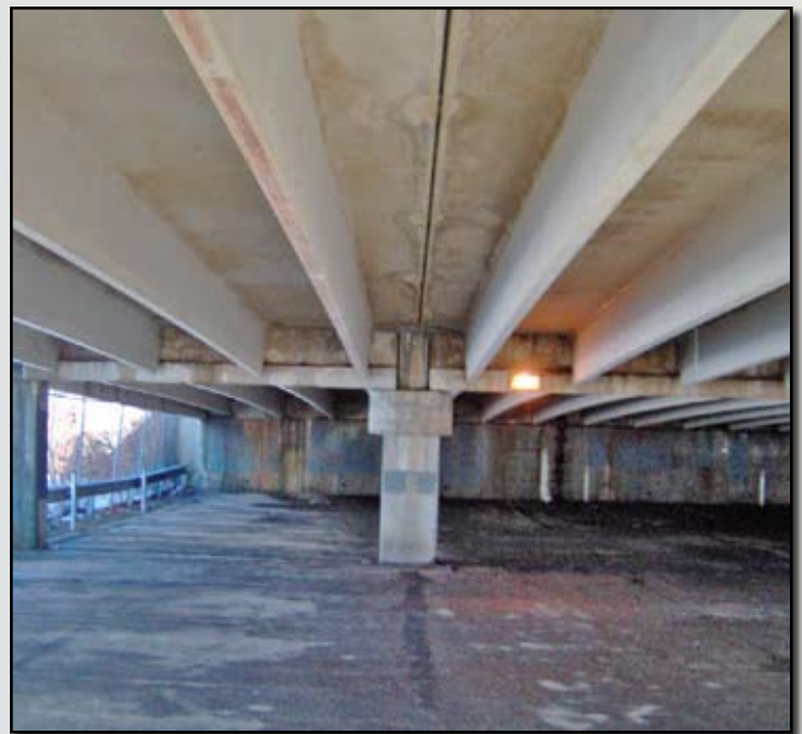
Underside of parking deck
