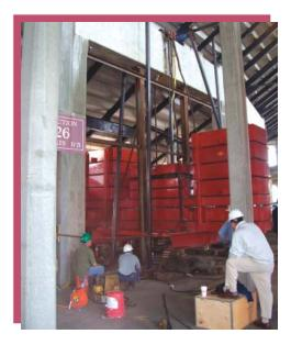
ACI 20.3.2. However, with the addition of supplemental beams and columns in 1982, the total test load requirement for the subject beam is reduced to 90 kips.
