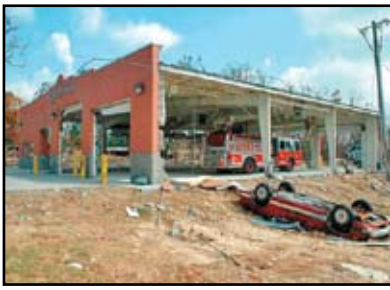
Figure 3: Storm Surge Damage, Gulfport, MS
