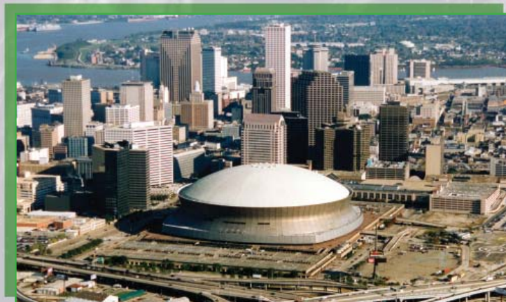
Superdome, New Orleans, LA. Photo courtesy of Walter P. Moore. Troy Gomez Photography©
