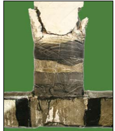
Figure 3: The failure of the beam column due to hinge formation in the beam section of the connection
