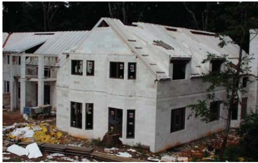
AAC Masonry building under construction
