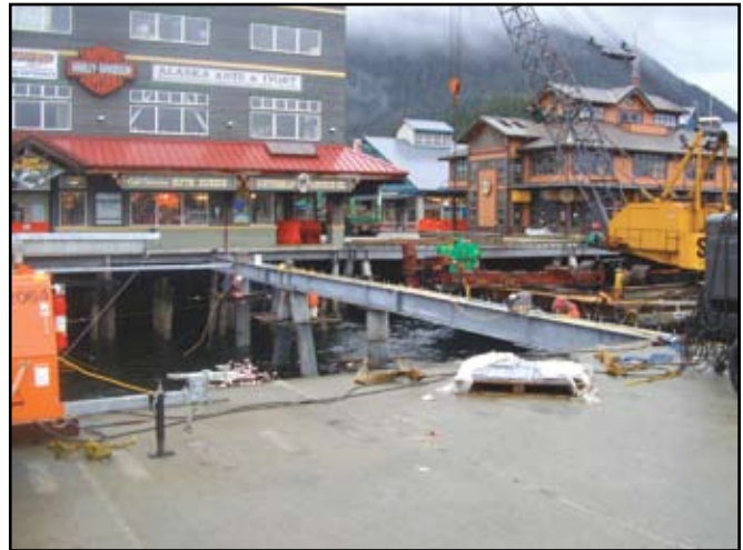
Spruce mill dock replacement during construction
