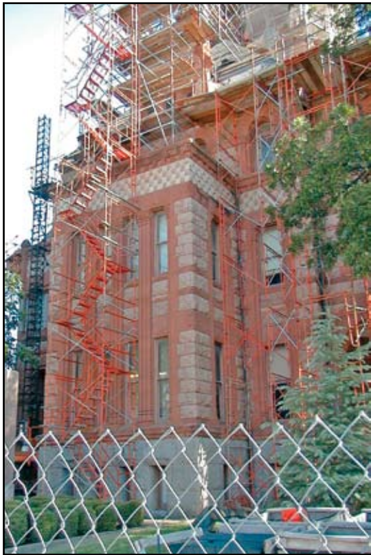
Exterior south stairs scaffolding, Ellis County Courthouse
