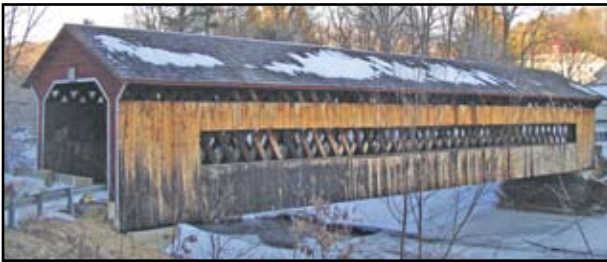
Figure 1: Winter setting of the covered bridge.
