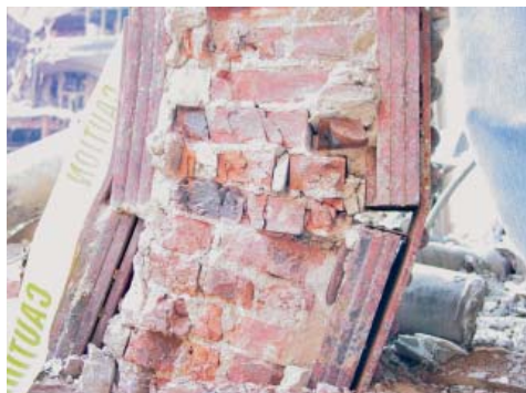
Figure 5: Column encasement preventing collapse
