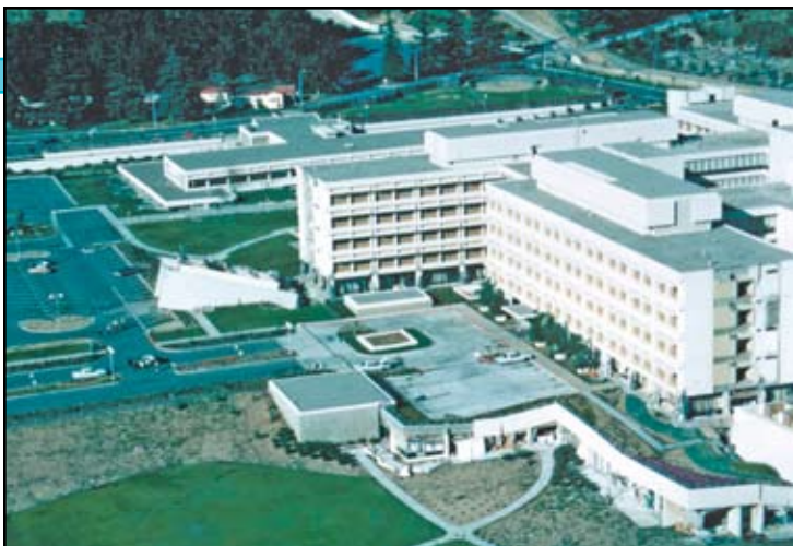
San Fernando, California, Earthquake February 1971. Two fallen structurally-separated stair towers and the collapsed basement at Olive View Hospital. View is north. Photo courtesy of USGS photographic archive.
