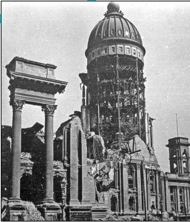
San Francisco, California Earthquake, April 18, 1906. View showing damage to the San Francisco City Hall. Photo courtesy of USGS Photographic Archive
