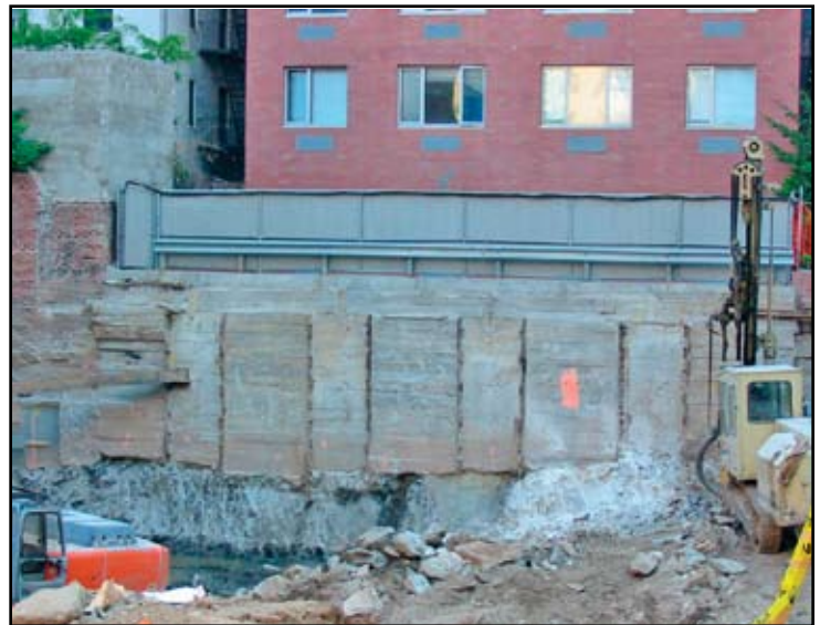
Figure 4: Completed concrete underpinning.
