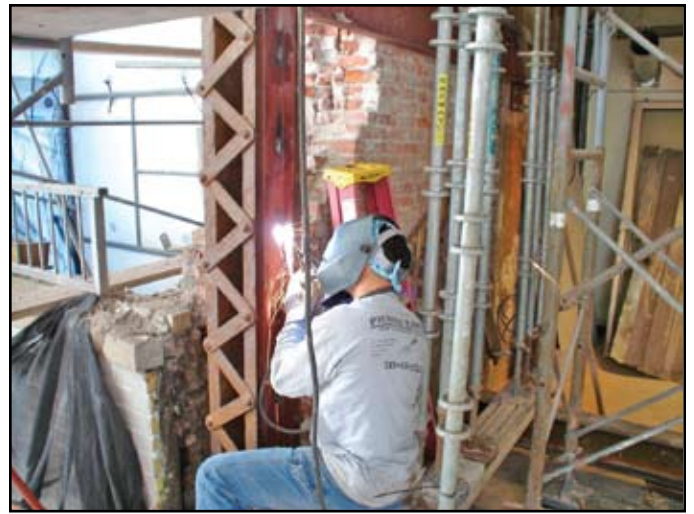
View of the column cutting during column removal
