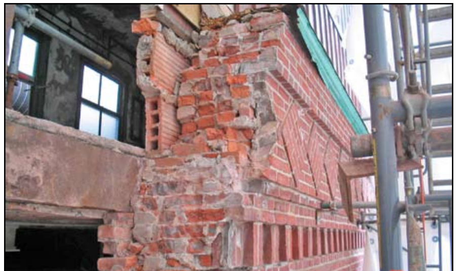
View of flat masonry arch and parapet
