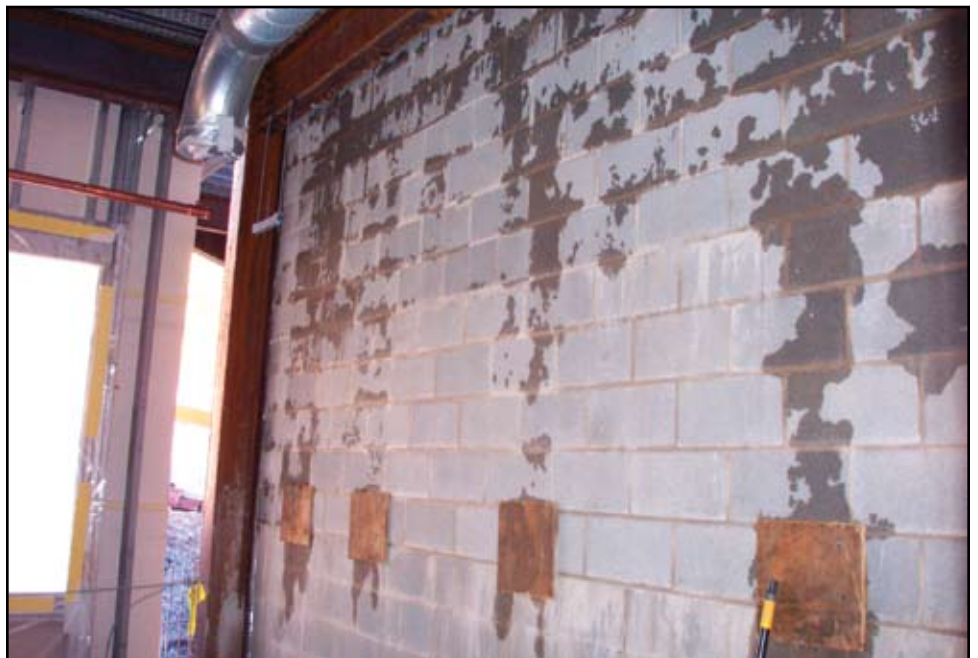
Freshly Grouted Wall with Cleanouts.
