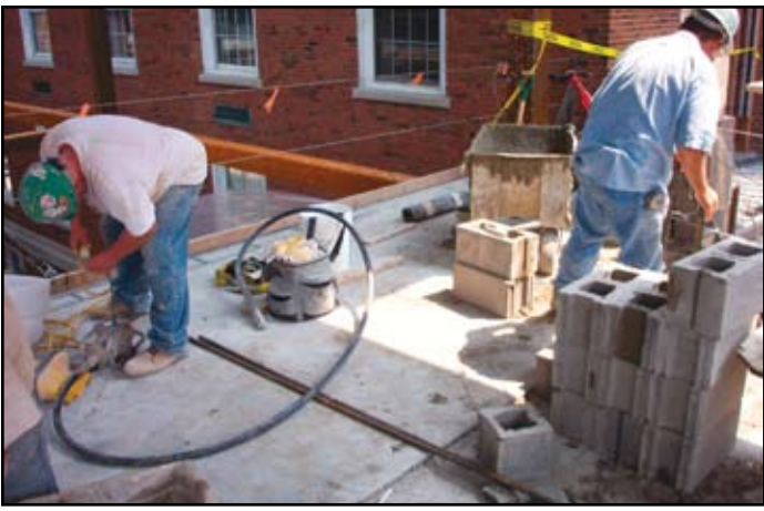
Pencil Vibrator for Grout Consolidation.
