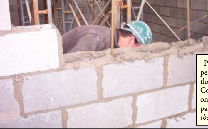
CMU Wall Under Construction.
