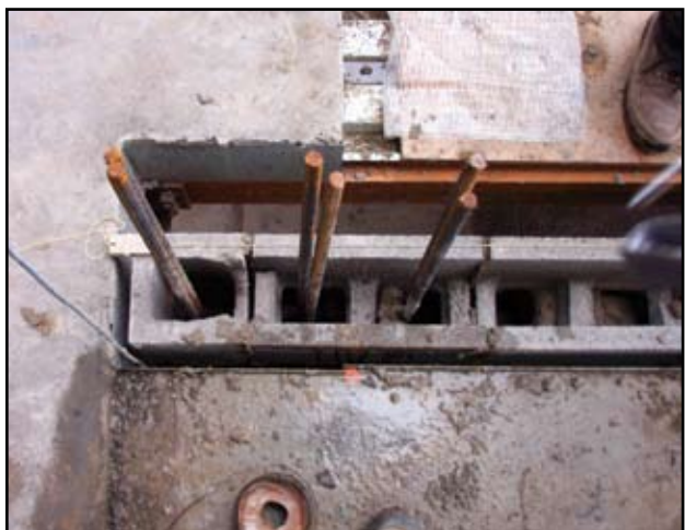
Heavily Reinforced Wall.
