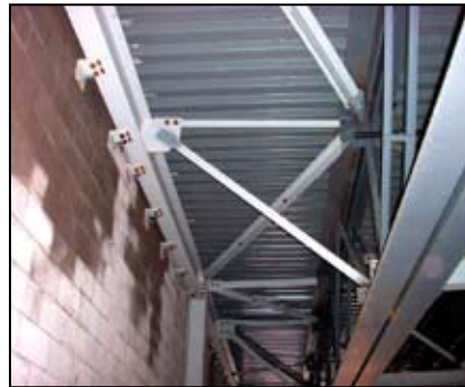
Steel roof framing with slotted clip connection to CMU wall
