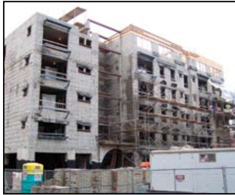
Six-story CMU bearing wall structure
