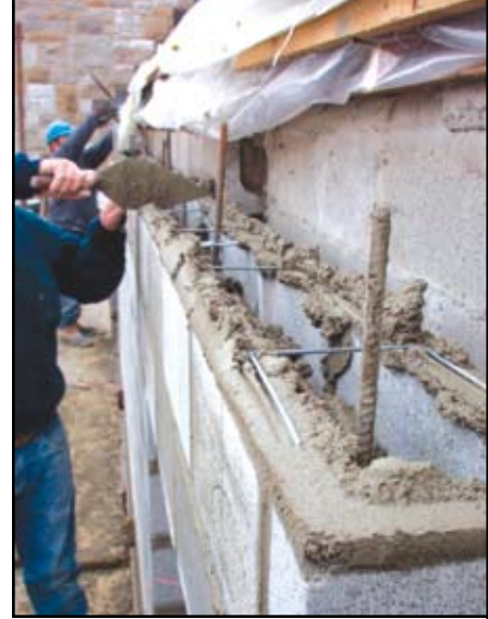
CMU bearing wall under construction
