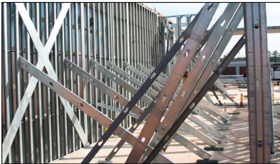
Figure 2: Construction Bracing during Installation.
