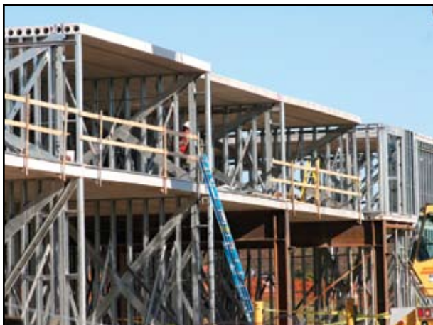
Figure 1: Vertical Alignment of Load Bearing Studs.
