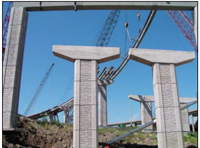
Figure 5: Similar aesthetic treatments decorate piers, abutments, MSE walls, and sound walls
