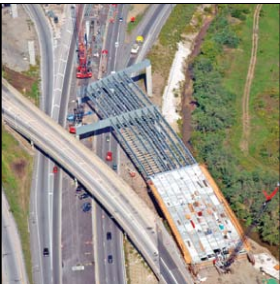
Figure 3: Construction of two steel capbeams over U.S. 71
