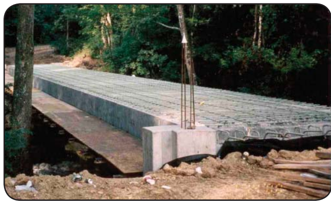
Deck ready to be poured
