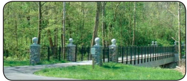
Side view looking southwest
