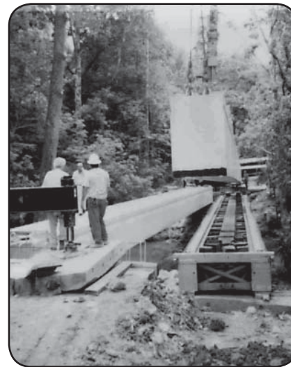
Prestressed beams being set
