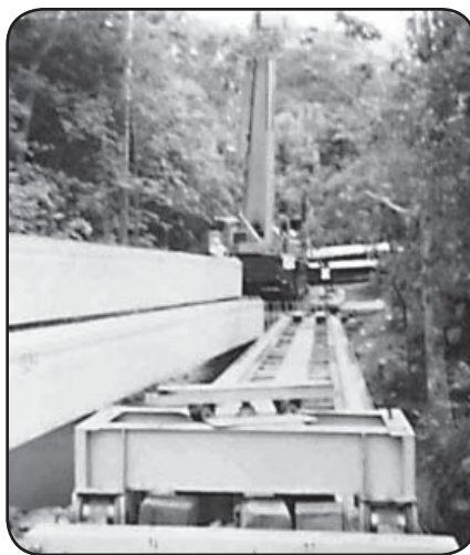
Spans being placed
