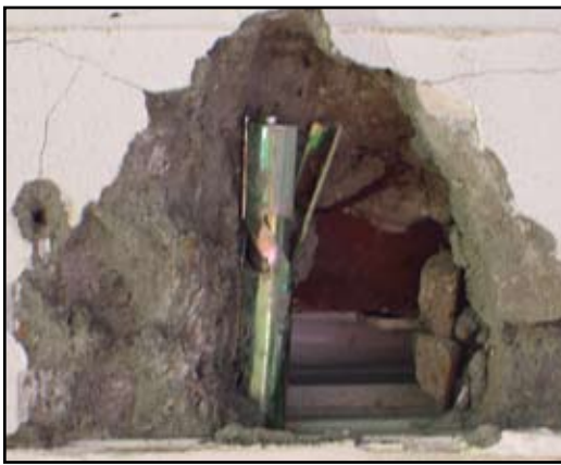
Substrate damage due to rotary percussion drilling.
