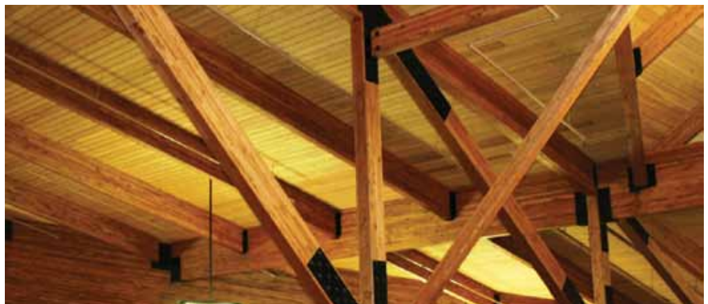
Glulam beams used in roof system.
