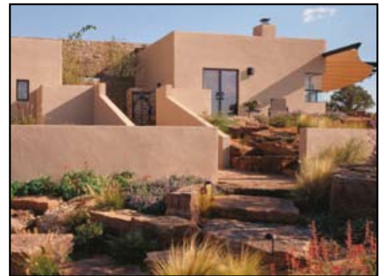
The design for this 7,550-square-foot home in Tesuque, New Mexico, created by Jon Dick with Archaeo Architects, is based on a traditional Mexican hacienda courtyard, but with contemporary detailing. The home features steel and fabric canopies on the exterior and a three-coat elastomeric stucco exterior finish.
