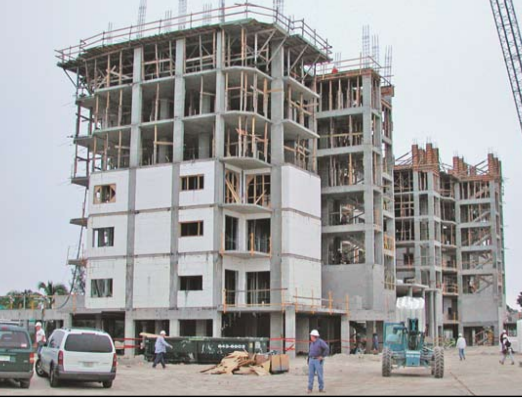
Construction of Waterside condominiums in Ft. Myers, Florida.
