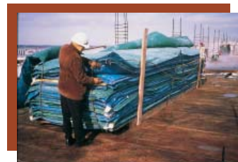
Figure 2: Insulating blankets for protection of concrete during cold weather
