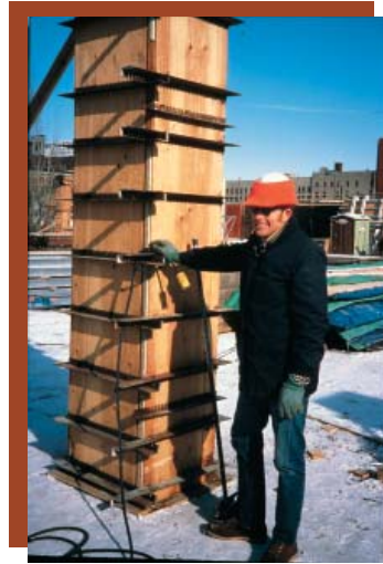
Figure 3: Insulated formwork for cold weather concrete protection
