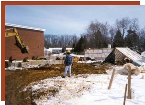
Figure 1: Cold-weather concreting protection using heated tents
