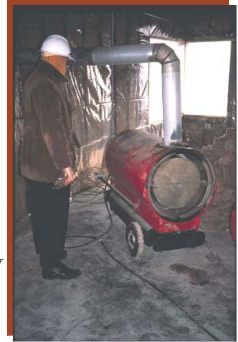
Figure 4: Cold-weather concreting protection with heated enclosures that are vented
