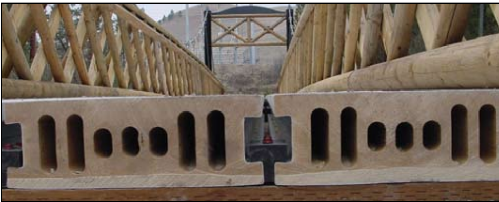
Figure 2b: Ribbed box sections (4x12-inches.) of PVC composite bridge decking.
