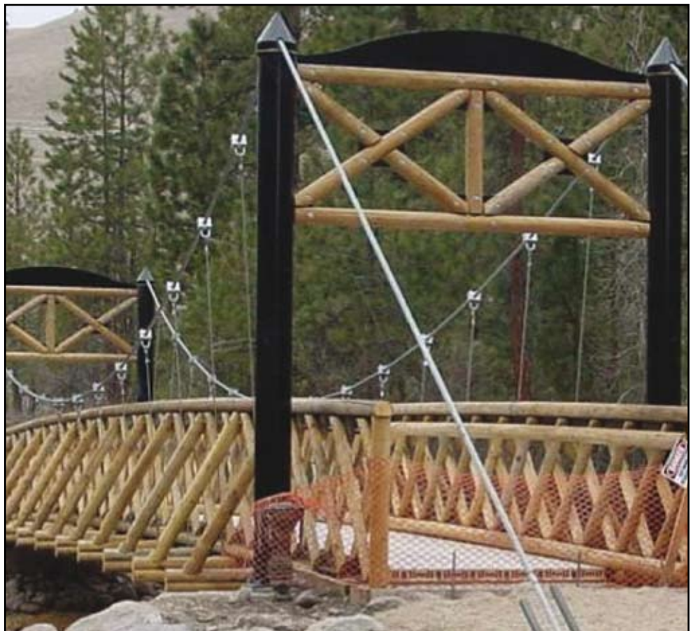
Figure 2a: Rattlesnake Bridge in Missoula, MT demonstrating WPC decking and small diameter round timbers.
