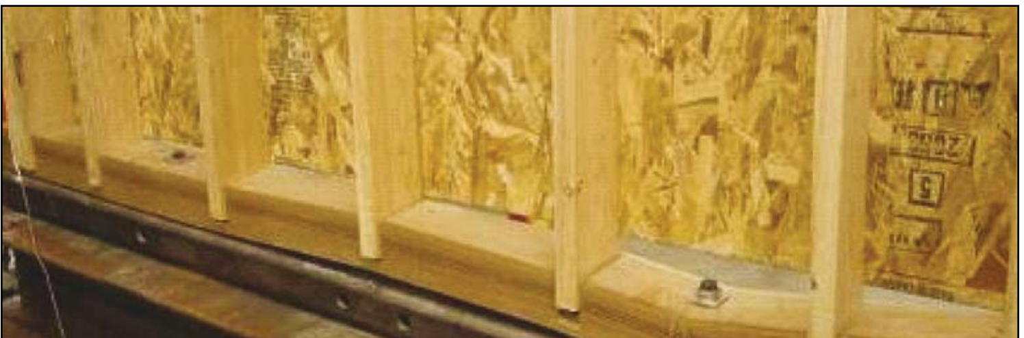
Figure 3. Test of braced wall panel using WPC sill plate.
