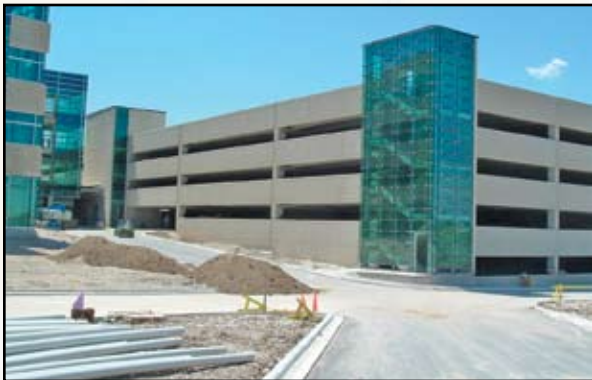
A 270,000-square-foot, four-level parking structure in suburban Milwaukee uses carbon fiber reinforced double tees
