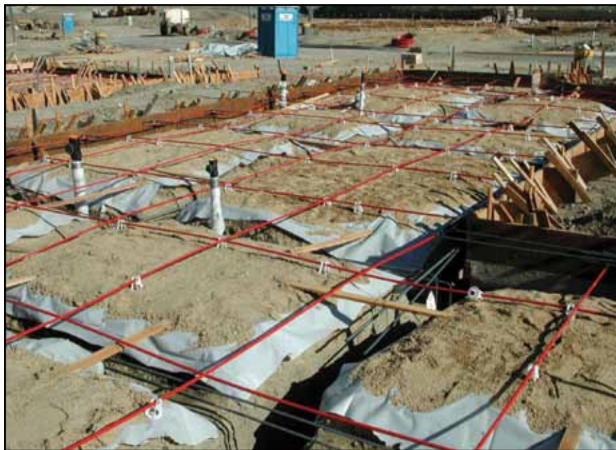
Figure 1: Ribbed Post-Tensioned Foundation.
