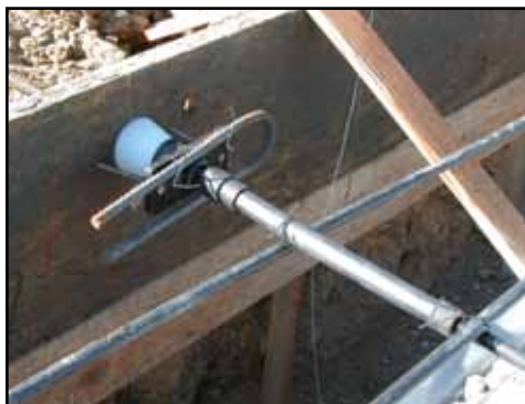
Figure 3: Encapsulated Tendon with a Pocket Former.
