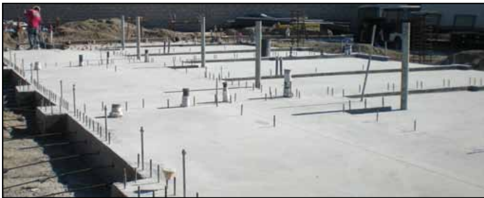
Figure 4: Saw Cuts on a Uniform Thickness Foundation.
