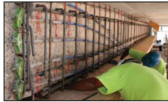
Completing surface preparation, steel/dowel placement and PT placement.
