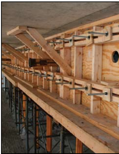
Form-and-pump formwork set for SCC pumping.
