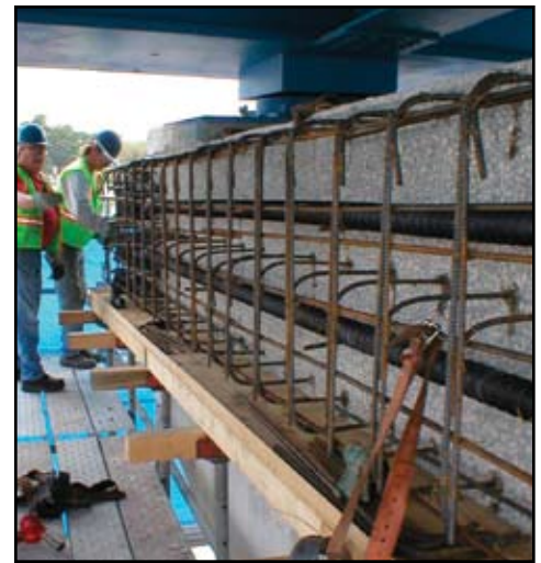
New post-tensioned enlargement on a bridge pier.
