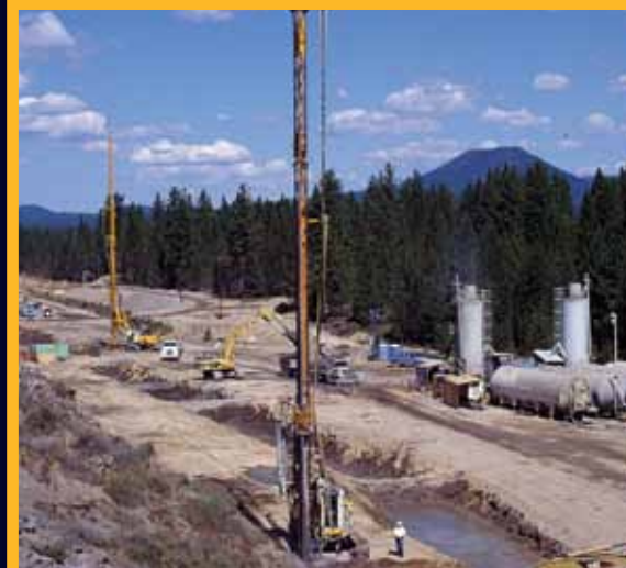
Compaction Grouting Harlem Hospital Center, New York, NY
