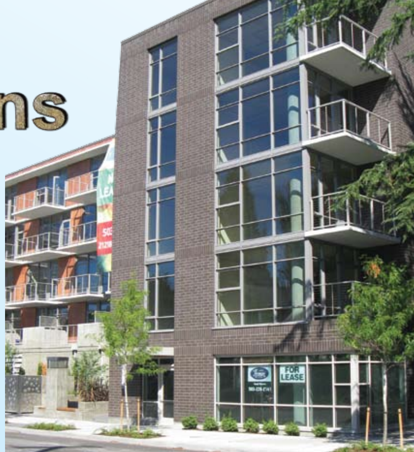
Figure 1: Finished building corner and exposed column that experienced soil settlement.
