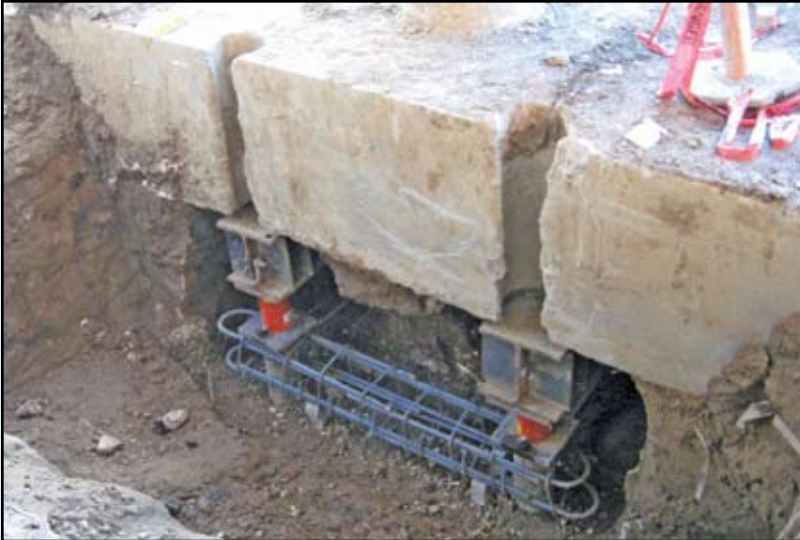
Figure 3: Reinforced concrete ties for the top of piles.
