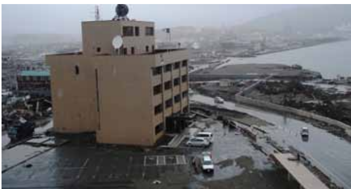
Figure 5: Kesennuma Port Authority Building. Courtesy of Ioan Nistor, ASCE.
