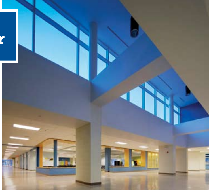
Figure 1: Clerestory windows. Courtesy of Wake County Public School System.
