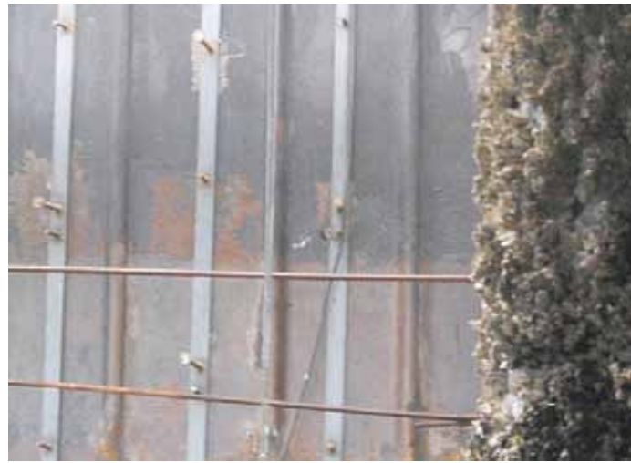
Figure 4: Pre-fabricated welded headed stud rails. Courtesy of Seaward Marine.
