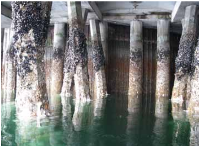
Figure 3: Existing concrete piers in close proximity to the cofferdam wall face.
