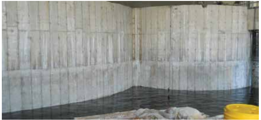
Figure 6: Completed cell and arc facing. Courtesy of Seaward Marine.
