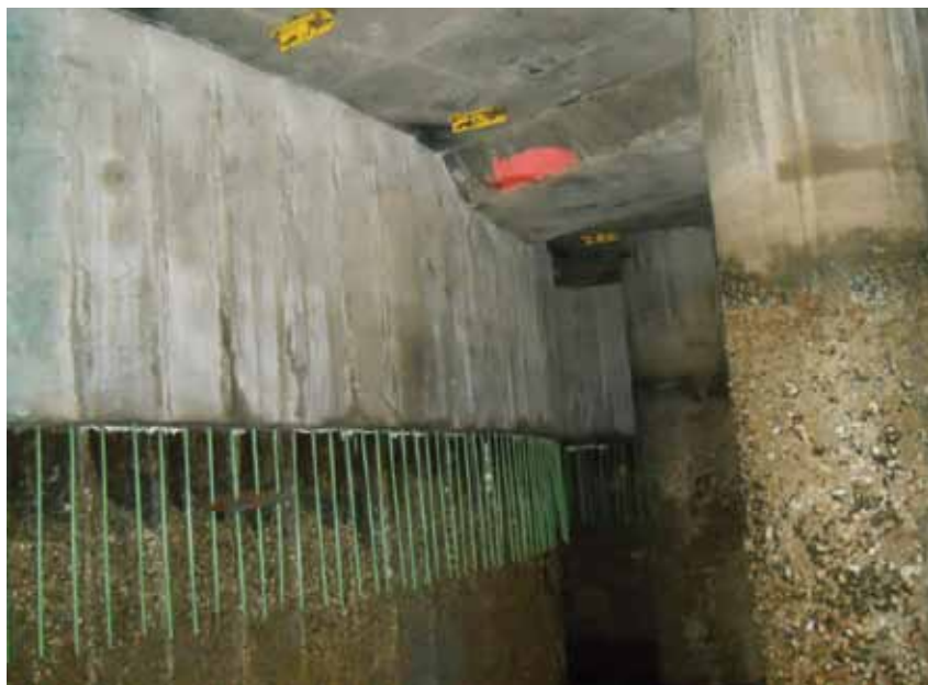
Figure 5: Completed "upper" facing under the pier. Courtesy of Seaward Marine.
