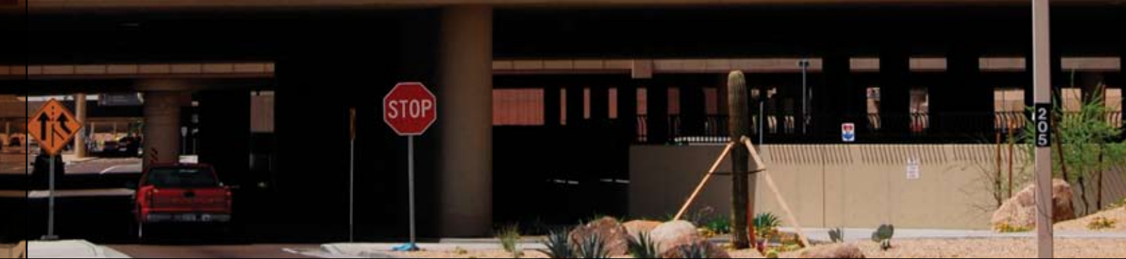
The new Taxiway Sierra Bridge at Sky Harbor International Airport in Phoenix. Courtesy of Richard Strange.
