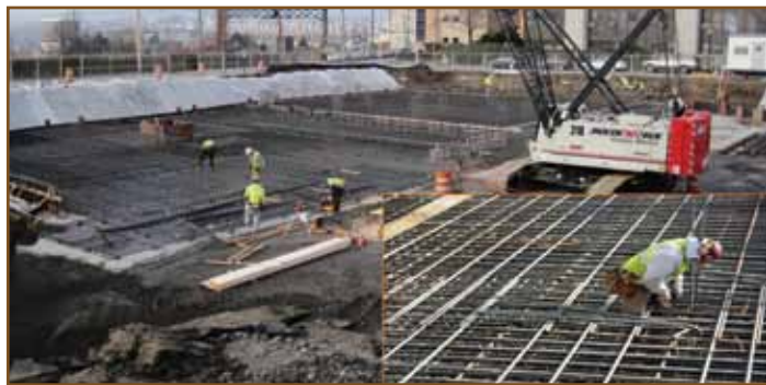
Mat Slab Foundation Construction.
