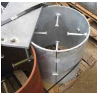
Figure 5: Steel collars prior to installation. The steel tab is visible at the bottom center of the photo. The collars were shipped with the internal bolts installed. These bolts were then removed, prior to placing the reinforcing cage, and reinstalled with the cage in place. The nuts that receive the bolts from the canopy framing members are also visible inside the collar.
