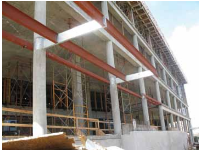
Figure 6: Steel collars installed in concrete columns.
