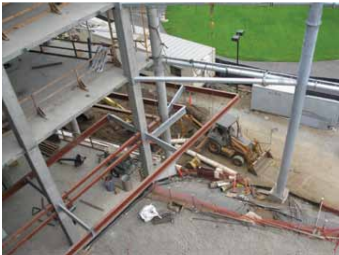
Figure 4: Canopy framing with bolted splices.
