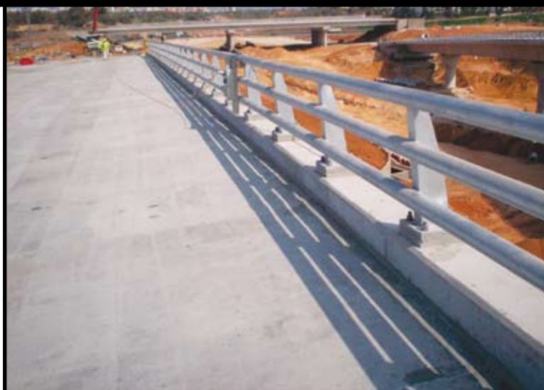
Ein Hakore Interchange, bridge construction completed ahead of roadway.
