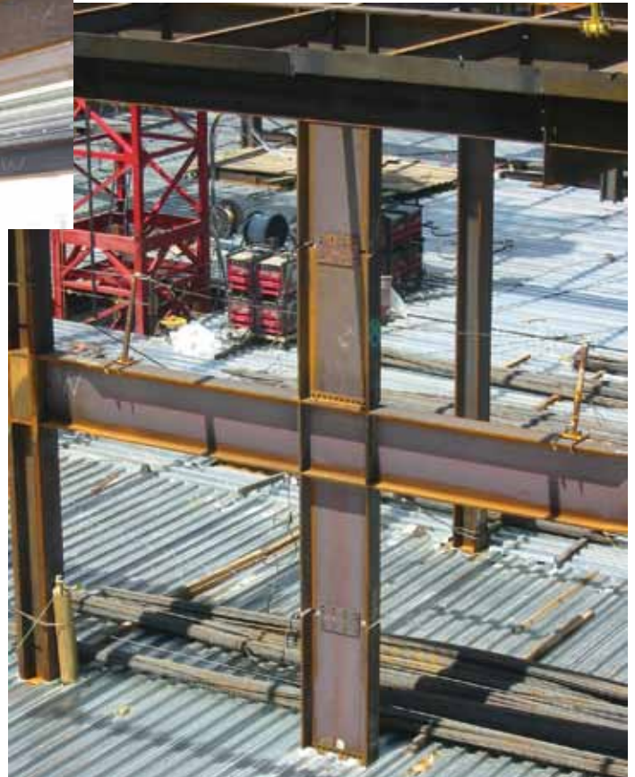
Shear links were added at the transfer levels to add stiffness to the structure.
