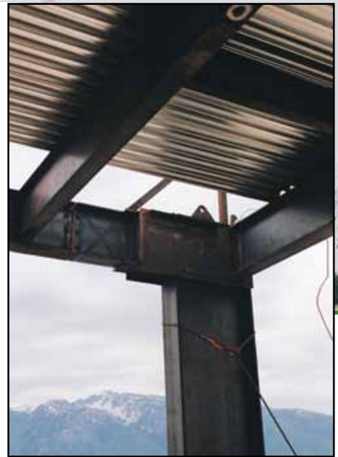
Corner SidePlate™ connection at roof.
