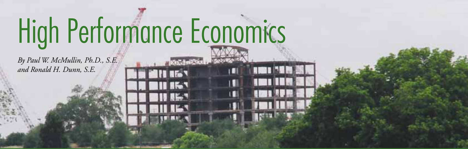
South elevation showing steel framing and interior shear walls.
