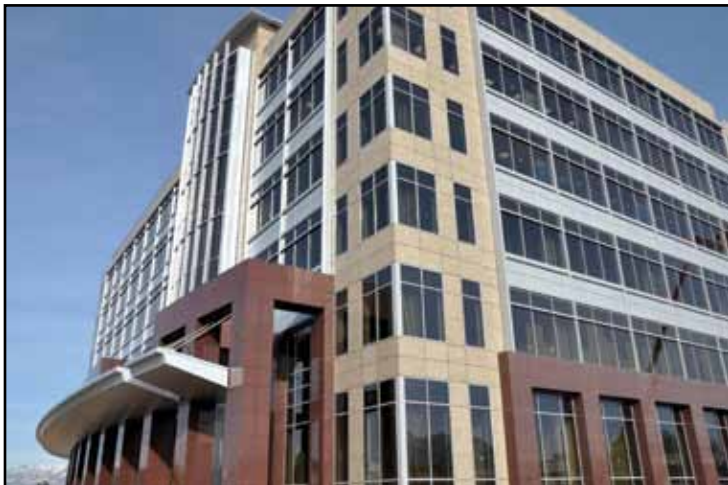
Finished, southeast elevation.
