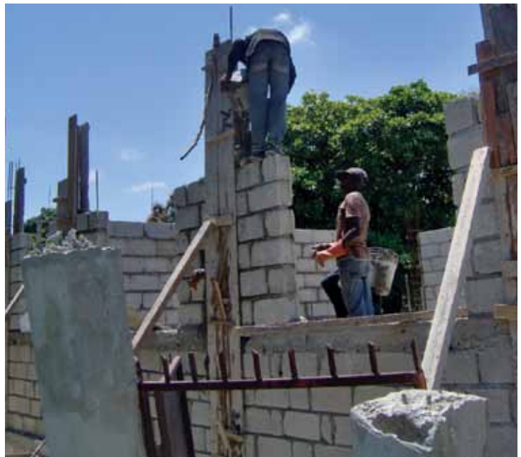
Pouring a Concrete Column Between CMU Walls.
