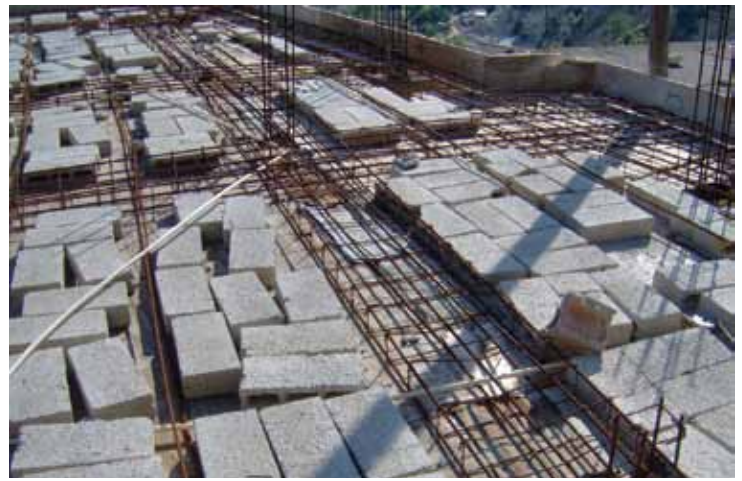
Typical Rib/Beam Slab Before Concrete Placement.
