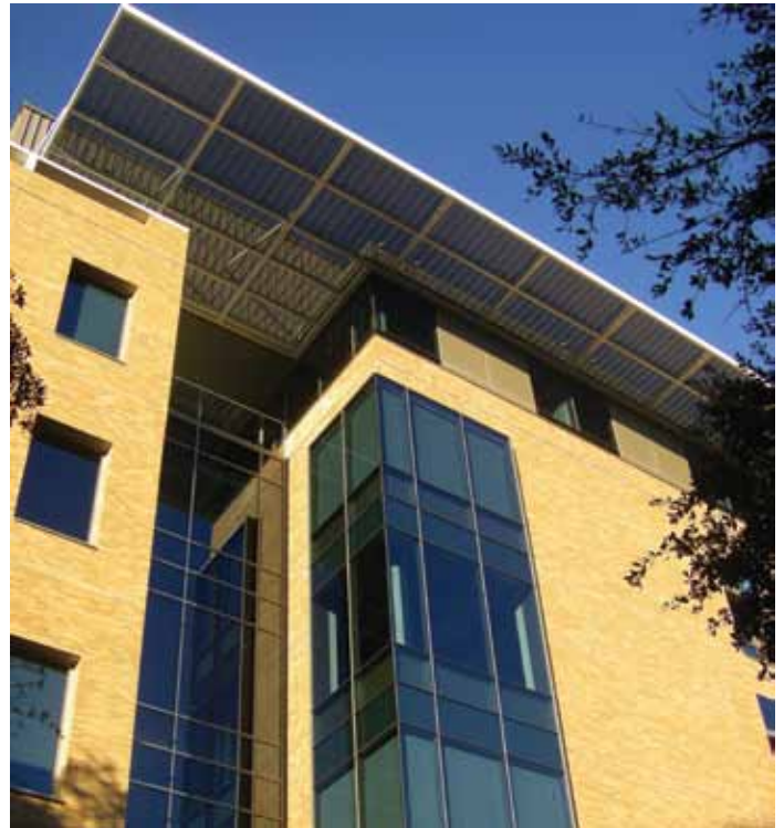
The setback at the west entry afforded an opportunity to conceal the expansion joint in a re-entrant corner.
