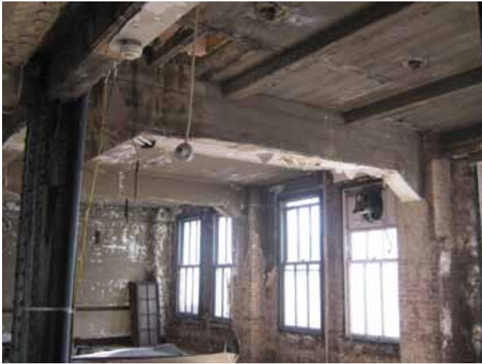
Figure 5: Existing encased bent prior to renovations.
