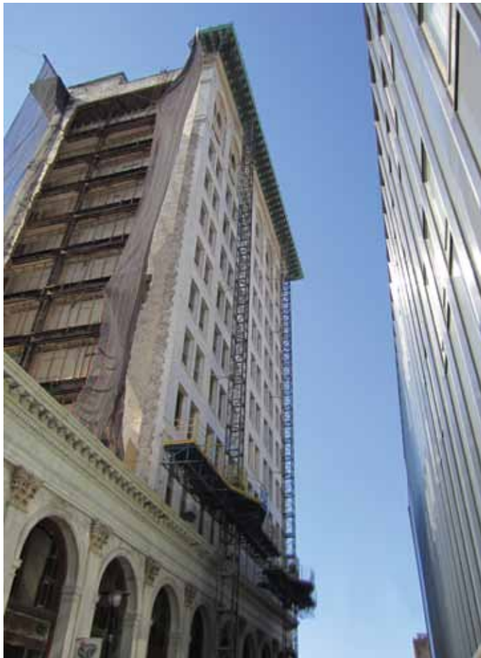
Figure 2: Exposed existing spandrels after east masonry wall demo.
