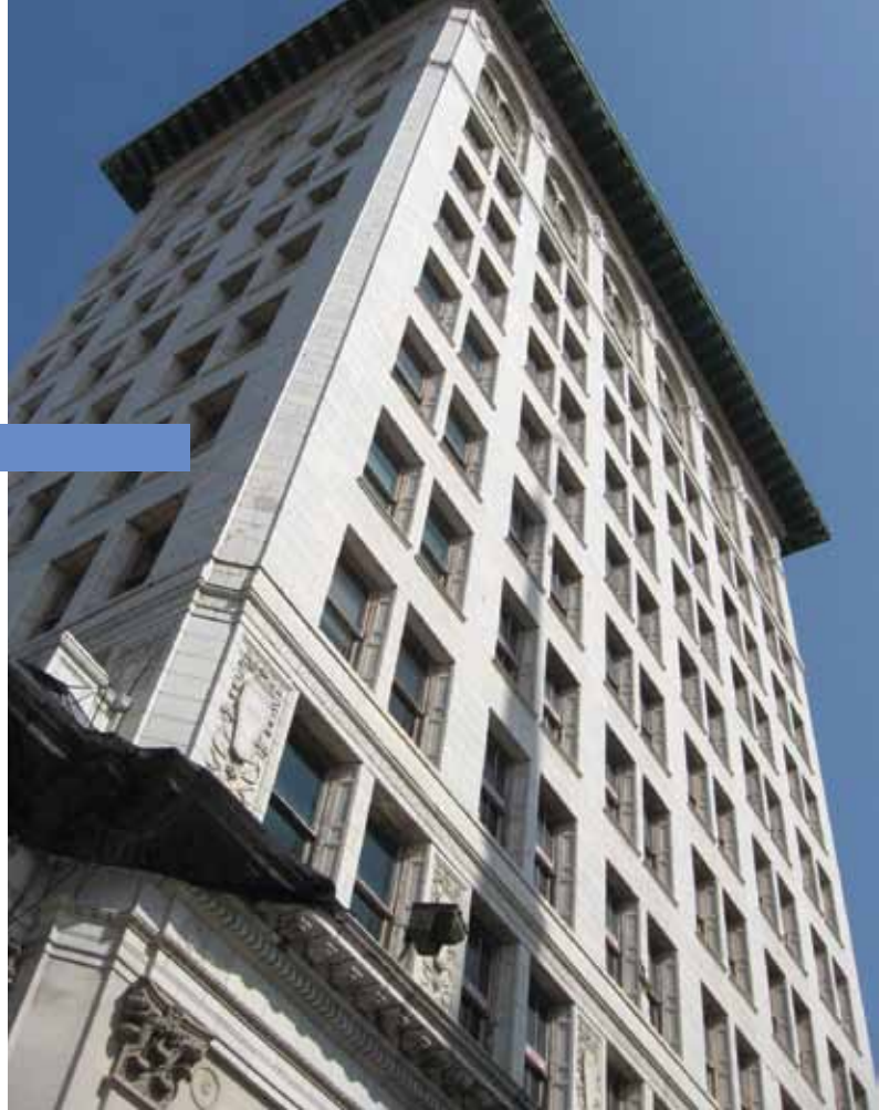
Figure 1: Existing façade prior to renovations.
