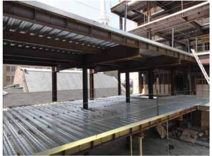
Figure 6: 4 th & 5 th floor addition north elevation cantilevers.
