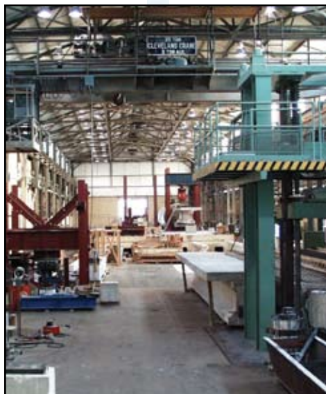
Figure 2: Main 400 foot long crane bay of FSEL.
