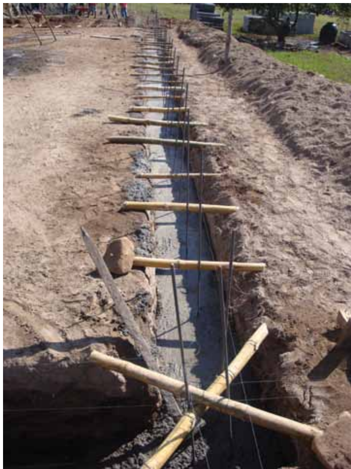
Figure 2: Reinforced Concrete Footings With CMU Dowels.
