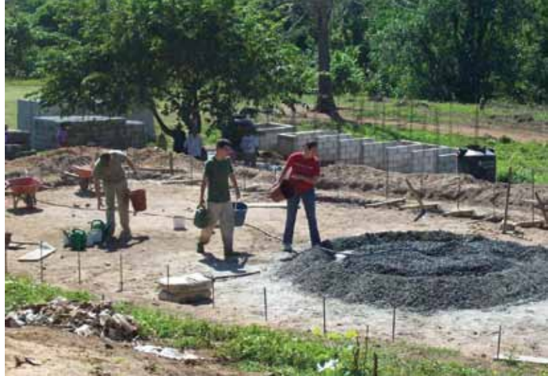
Figure 1: Local Method for Mixing Concrete and Water Distribution.
