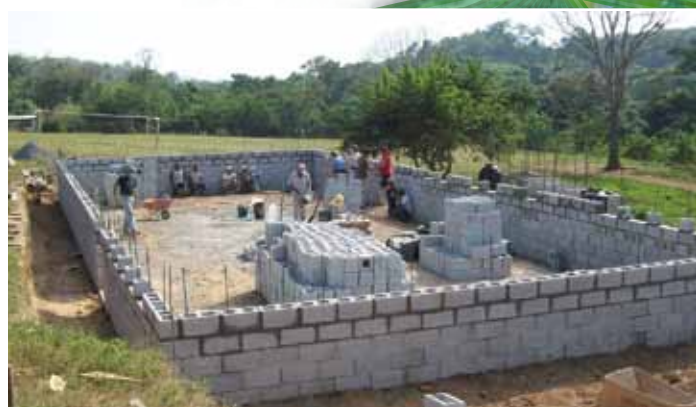
The School Building with Walls Erected Up to Midspan.
