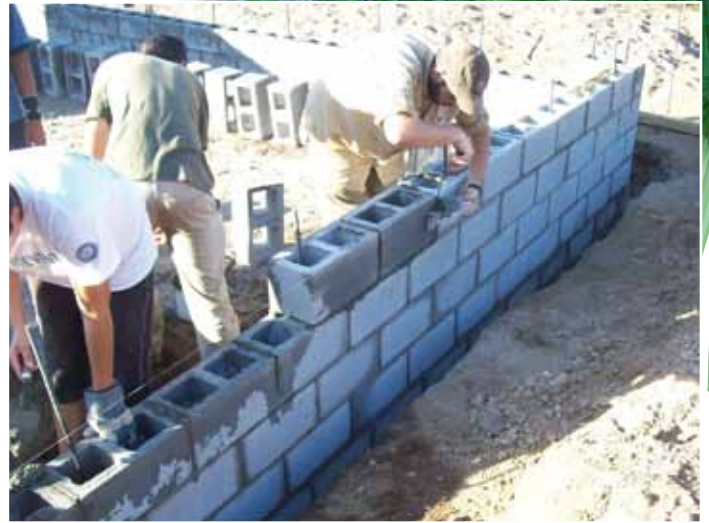
Figure 4: Working Off a Corner, Placing Block and Pointing Joints.
