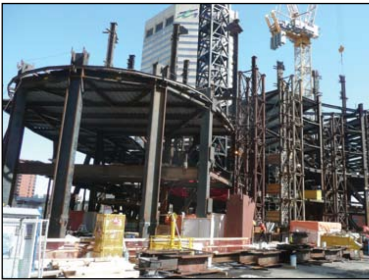
Figure 6: Photo of Atrium Wall.
