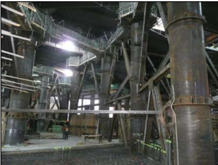
Figure 4: 'Top-Down' Construction Techniques.
