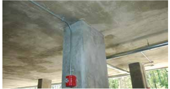
Slab-column joint at First Level near northwest corner of slab.
