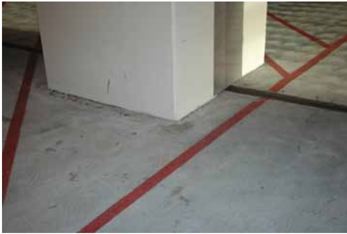
Figure 4: Same Location as Figure 3, One Floor Up On Level L2.
