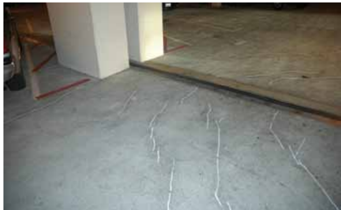
Figure 3: Top of slab near expansion joint, structure A2 Level L1.
