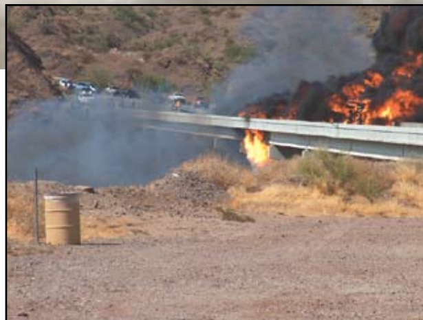
July 28, 2006 Fire – Looking North at West Side of Concrete Bridge. Courtesy of Bill Williams National Wildlife Refuge, U.S. Fish and Wildlife Service.
