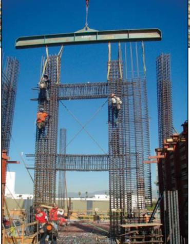
Shear wall rebar was detailed to allow pre-tying of cages offsite. This minimized field labor and accelerated construction.
