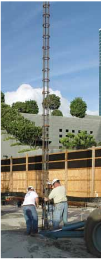
Figure 2: Pilot Hole Drilling.
