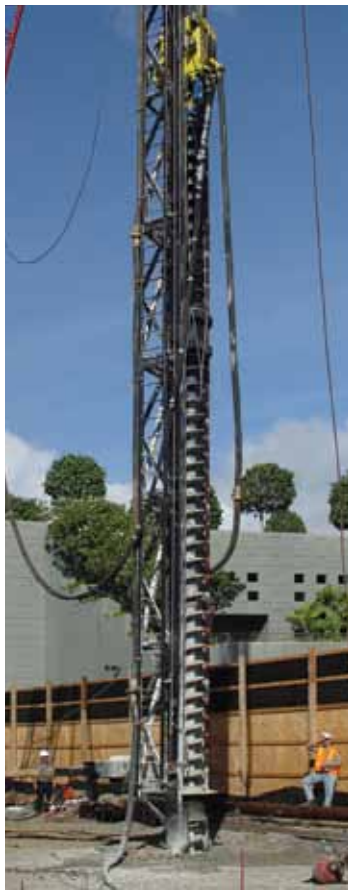
Figure 3: Installation of Reinforcing Cage.
