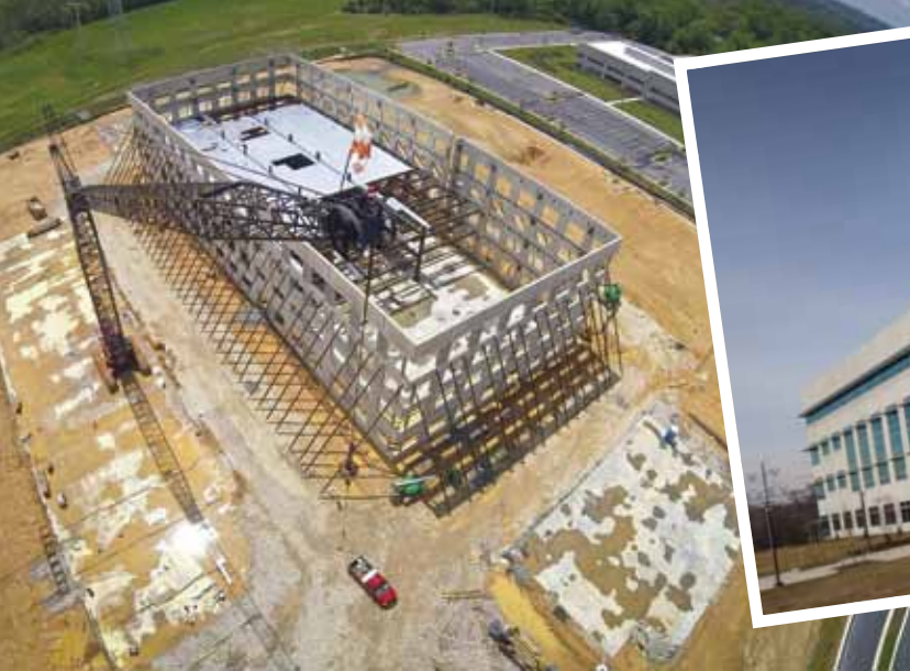
Aerial view of steel erection in progress.
