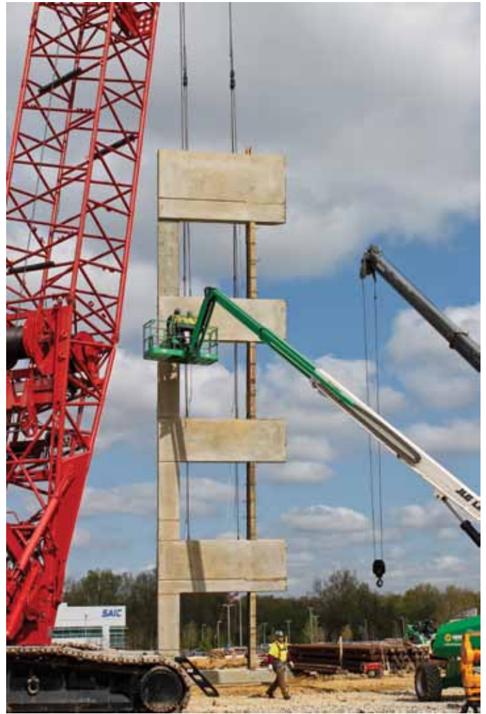
Erection of corner panel with strongbacks.
