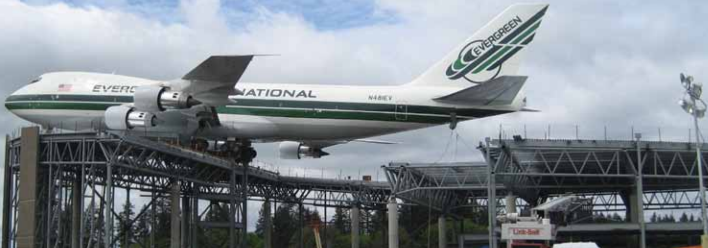
The plane in its final position on the roof of the partially completed structure. Courtesy of Jeffrey Diephuis.
